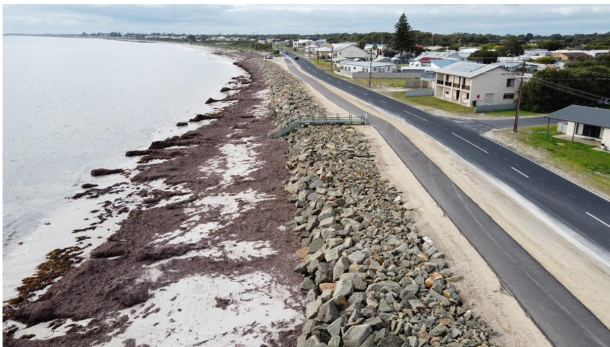
Figure 20. Wyomi Beach, Kingston SE, sea wall and nourishment sand in 06-07-2020. (P. Hesp Photograph).
