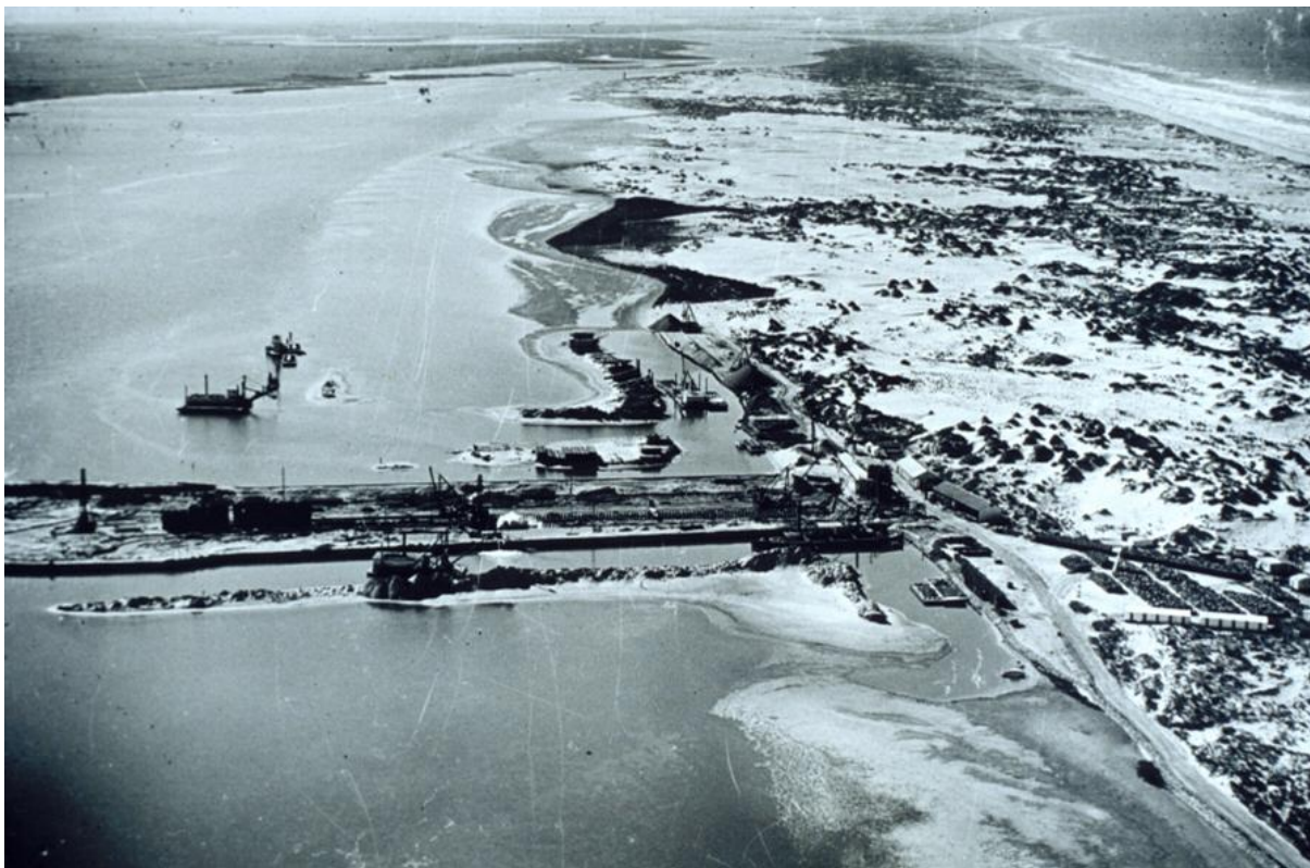
Figure 24. An overview of the Sir Richard Peninsula during the construction of the Goolwa barrage some time between 1933 and 1937 (D. Darian Smith photographer). Image BRG 397/2/114A/5 courtesy State Library, SA. View is down River towards the Murray Mouth.
