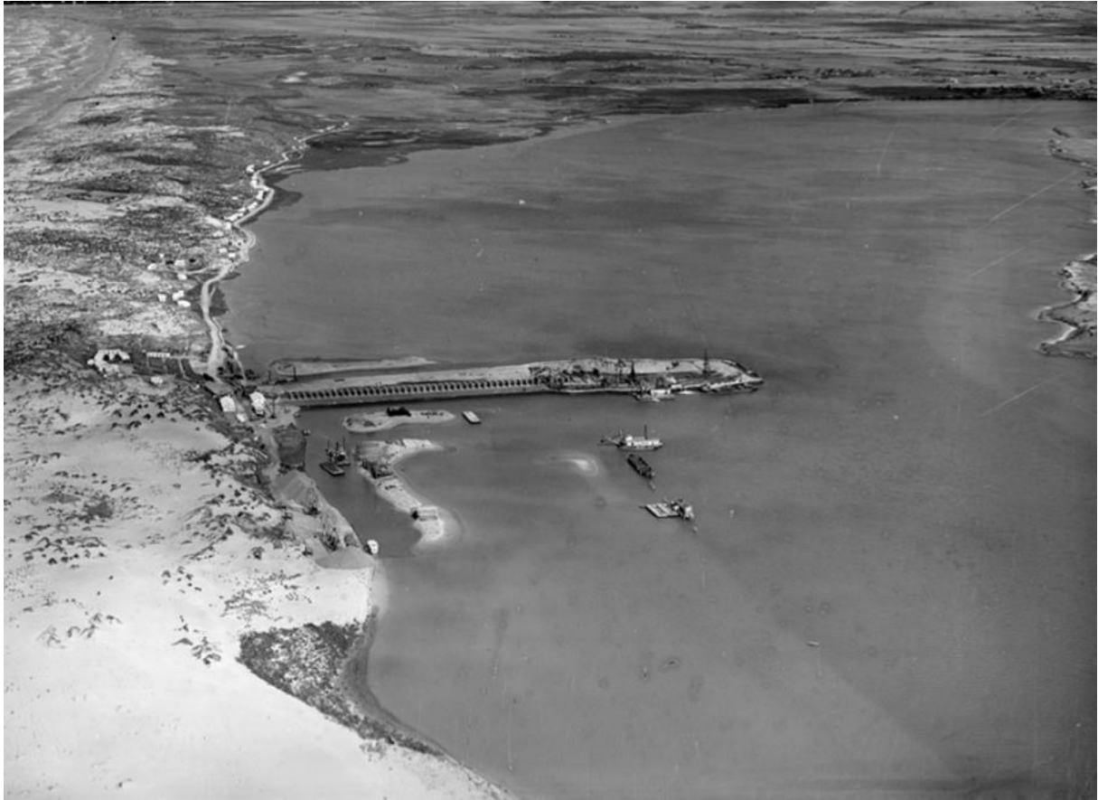
Figure 25. Image looking up River of the Goolwa barrage being built some time between 1933 and 1937 (D. Darian Smith photographer). Image BRG 397/2/114A/2 courtesy State Library, SA.
