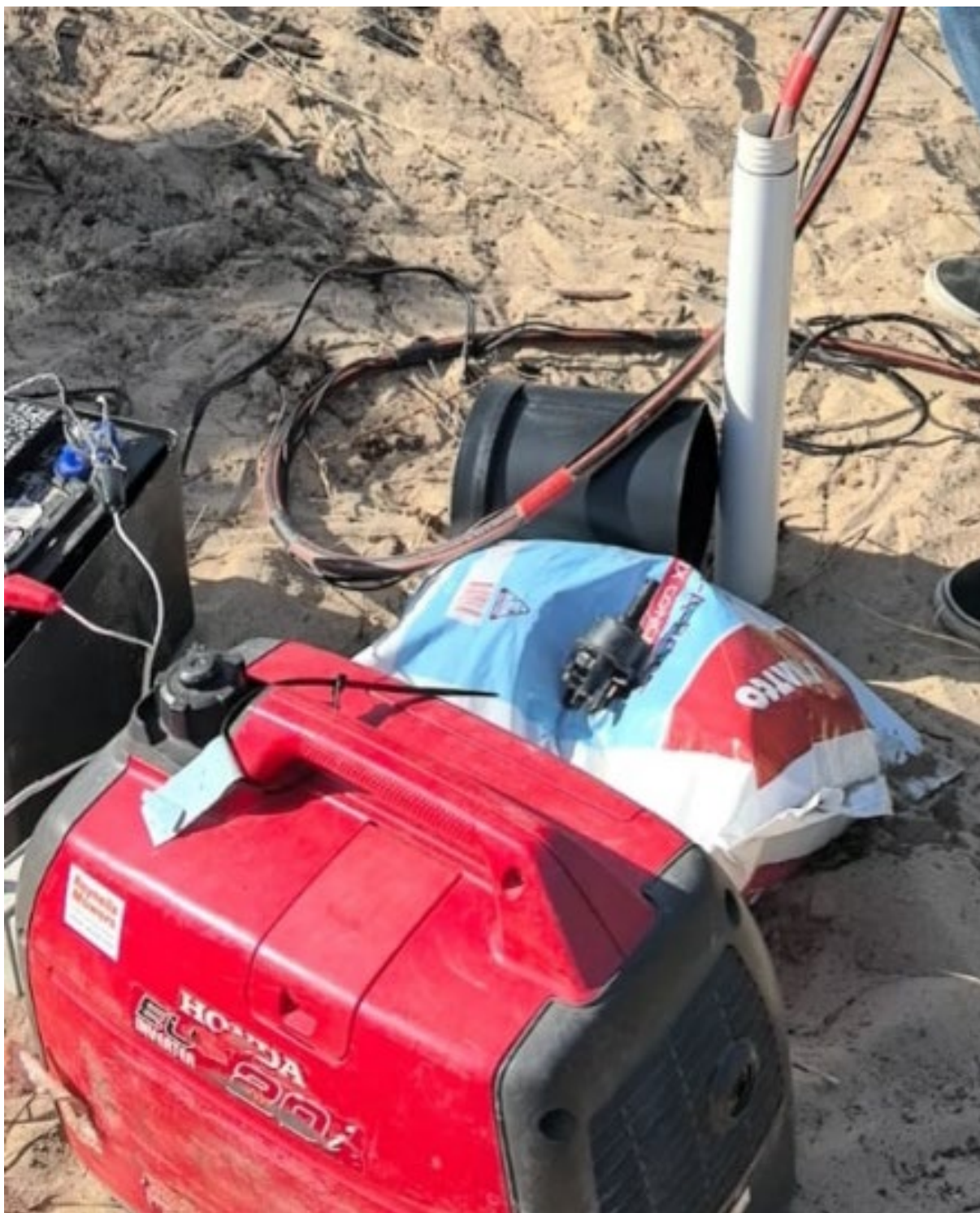
Figure 15. Pumping groundwater from Well 2 (Photo credit: Guohua Hou taken on 13 October 2025).
