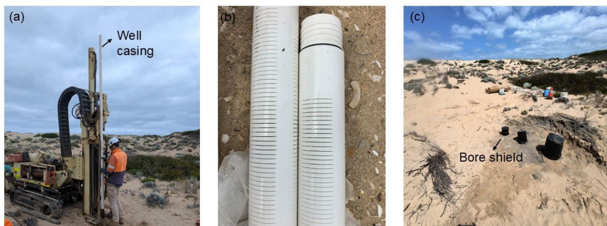
Figure 6. (a) Installation of well casing, (b) Screened section of well and (c) Bore shields at Site 5 (Photo credit: (a) Sanjukta Das taken on 7 October 2025, (b) and (c) Guohua Hou taken on 10 October 2025).
