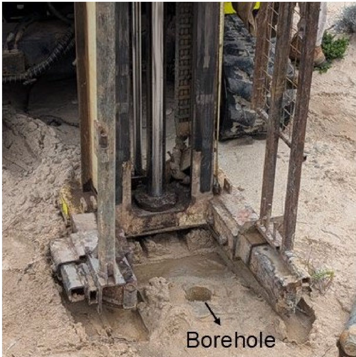
Figure 4. Borehole 5C drilled at Site 5 (Photo credit: Sanjukta Das taken on 7 October 2025).
