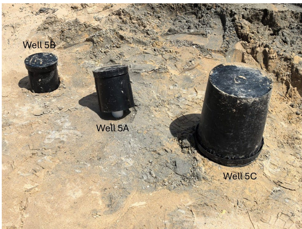
Figure 16. Wells 5A, 5B and 5C, prior to completion of the bore shields, etc. (Photo credit: Guohua Hou taken on 10 October 2025).
